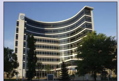
Three VHP7100 Enginators® and an APG1000 Enginator unit are powering the Northwest Community Hospital in Arlington Heights, Illinois.
